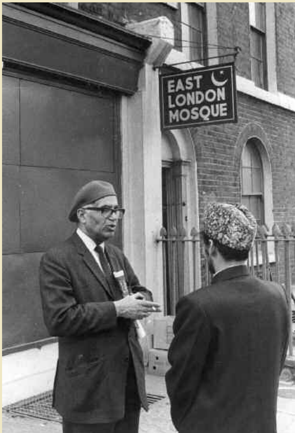
The site of the original East London Mosque in Commercial Road. 1972 © Tower Hamlets Local History Library and Archives
