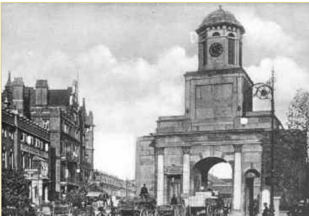
Entrance to East India Dock, 1912 © Tower Hamlets Local History Library and Archives
